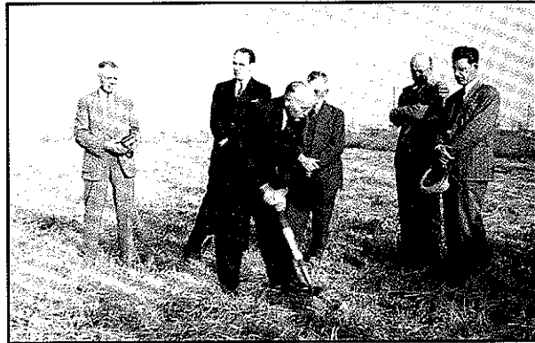
Blessings poured down abundantly from the Lord: the building site dedication May 4, 1941...Pastor Burandt's acceptance of the call...his installation September 21...and ground breaking in October:
