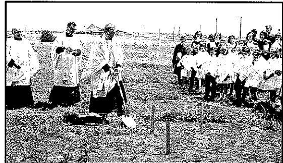
Site dedication and ground breaking for the John of Beverly Deaf Chapel, a Fellowship Hall, classrooms for the school and administrative facilities for the church staff were held on Easter Sunday, April 18, 1966.
